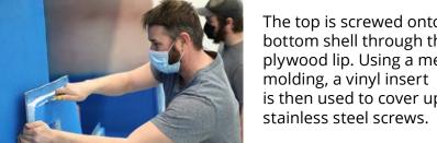
The top is screwed onto the bottom shell through this plywood lip. Using a metal is then used to cover up
